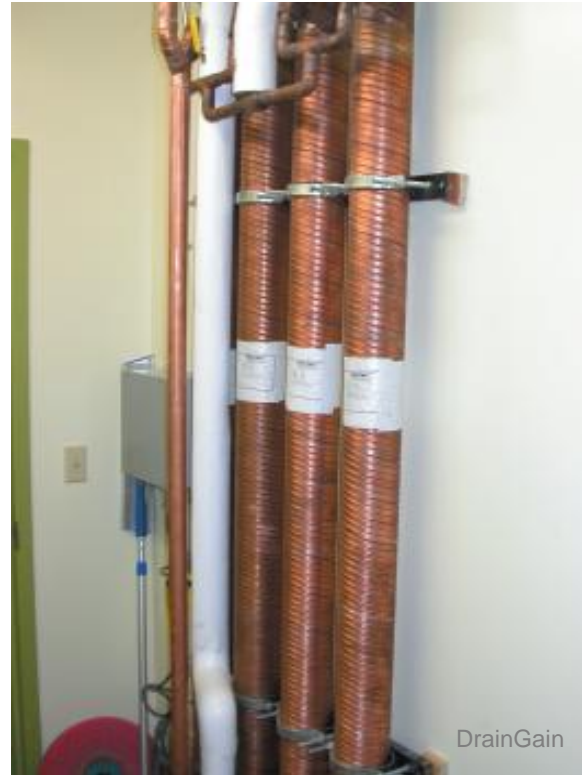
Système GFX Drain Water Heat Recovery System (DWHRS)
